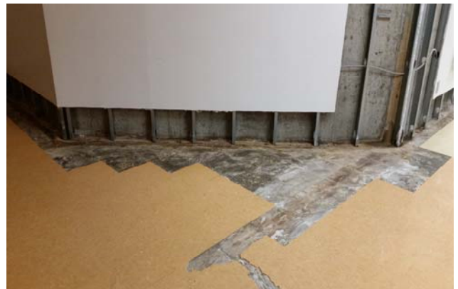
Below: Water seeping undetected underneath the tiled floor is exposed, showing damage that continues under the rest of the adjacent tile.
