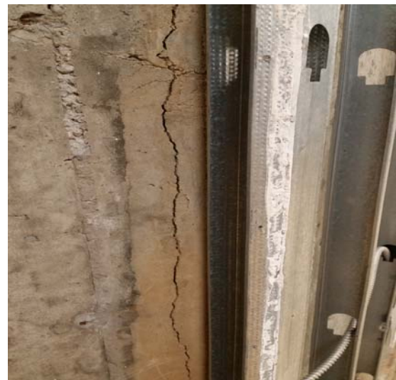
Above & Below: Two cracks in the foundation which run from the floor to the ceiling, leaving puddles of water on the floor.
