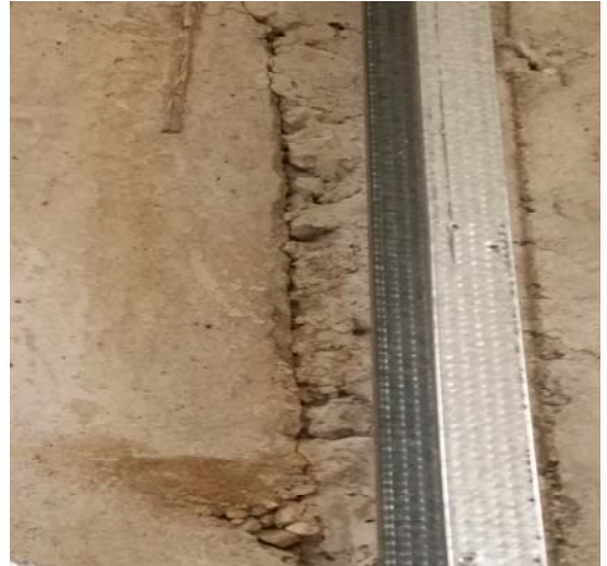
Above & Below: Two cracks in the foundation which run from the floor to the ceiling, leaving puddles of water on the floor.
